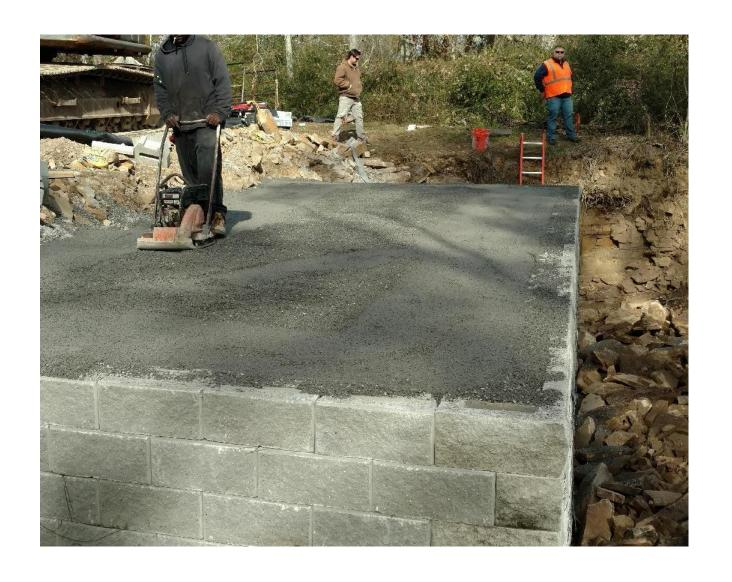
Abutment 1 15<sup>th</sup> Course Bearing bed reinforcement
