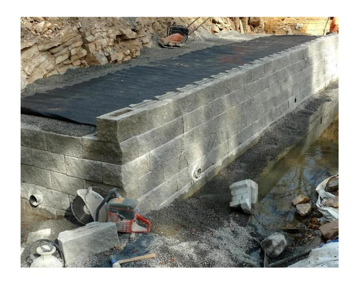
Abutment 1 Checking Line and Grade 6<sup>th</sup> Course(typical)
